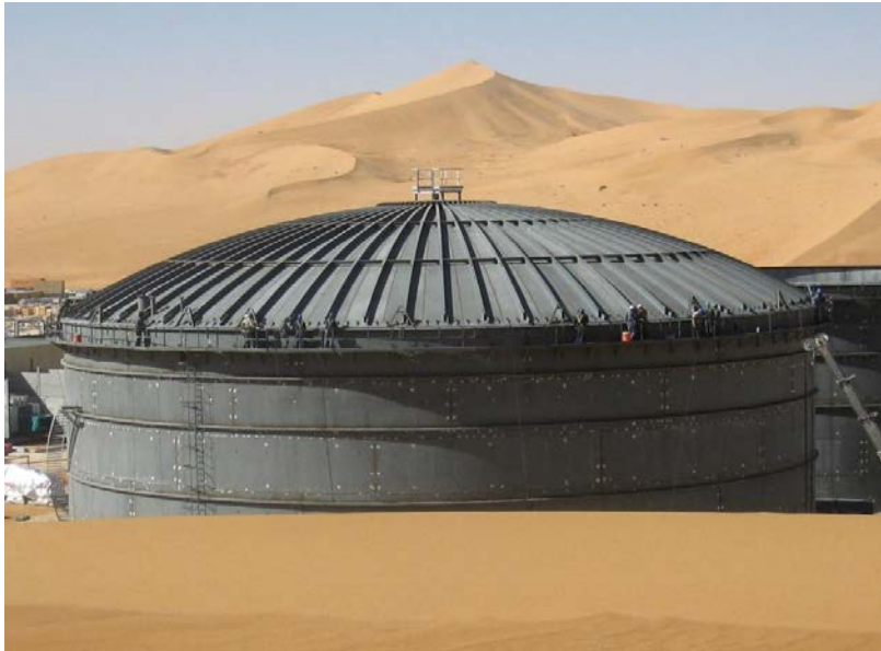
Fixed roof tanks
