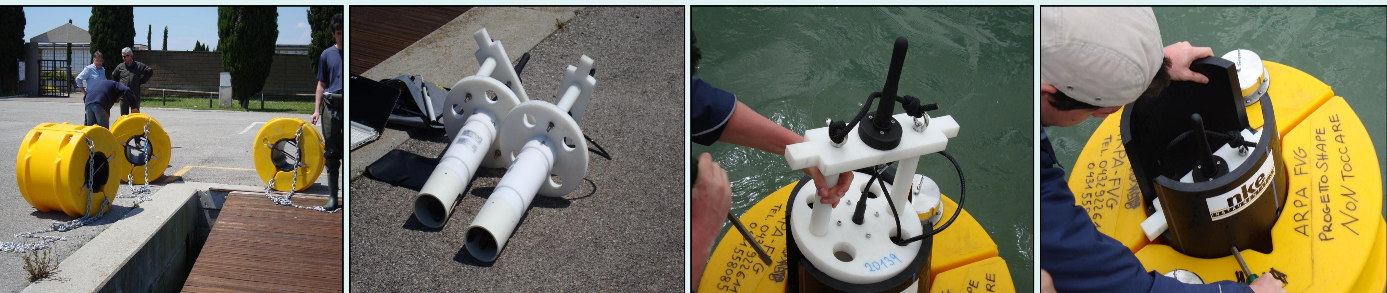
Fig.4 Some pictures of the installation of the instruments acquired by ARPA FVG with funds of the SHAPE project.
